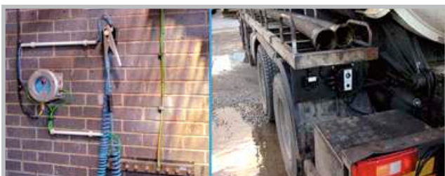
Figure 2: Examples of a gantry mounted (Earth-Rite® RTR) and tanker mounted (Earth-Rite® MGV) static ground verification systems.
